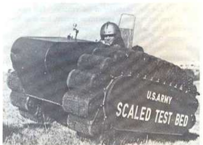
Fig. 1 - Four-tenths scale model test bed
