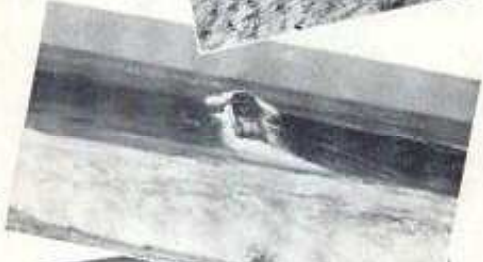
Soft sand and sand dunes are sought out at the Warren Dunes State Park on Lake Michigan to test tractability of the large low pressure tires. Results were excellent.
