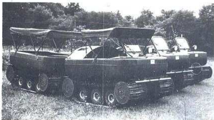
Fig. 12—"Dinah" light general-purpose tracked vehicle designed for operation in difficult terrain
